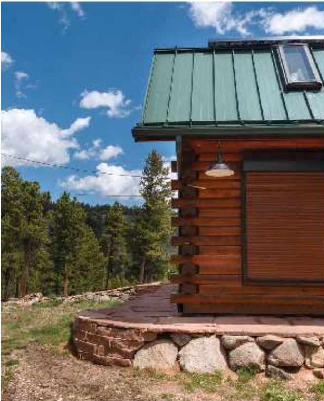
Bottom: A metal roof and noncombustible exterior window coverings add layers of protection against wildfire, in addition to the well-maintained defensible space that surrounds this home. Photo: Wildfire Partners
