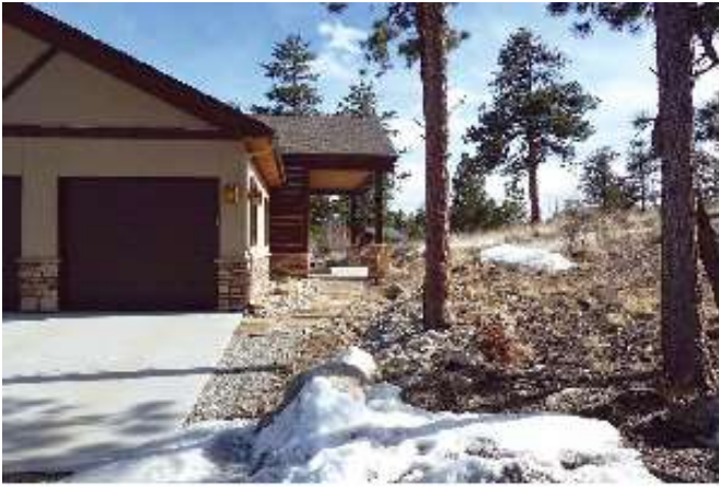
Top left: Hardening your home can include choosing noncombustible building materials like stucco paired with a stone facade. This house near Salida shows you don't have to sacrifice curb appeal to reduce the ignitability of your house. Photo: CSFS
